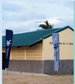
Rehabilitated classrooms – Inhassoro
